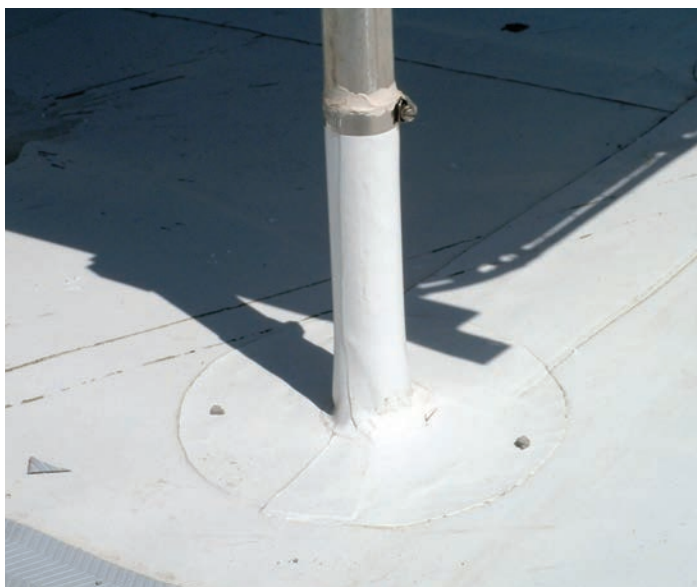
Flex Split Pipe Boot, a pre-fabricated flashing
