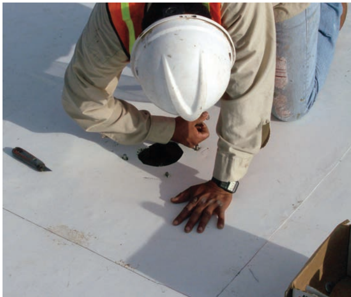
Installing a Flex TPO Flashing target sheet over the field sheet drain opening
