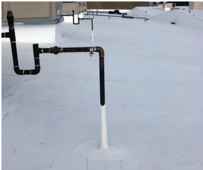
Field-fabricated method with Flex TPO Flashing Membrane
