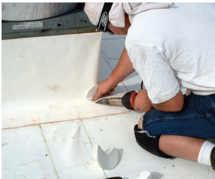
Hand welding a pre-formed outside corner flashing
