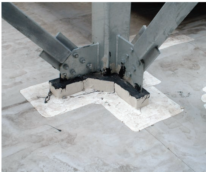
Pitch pans solve difficult flashing details
