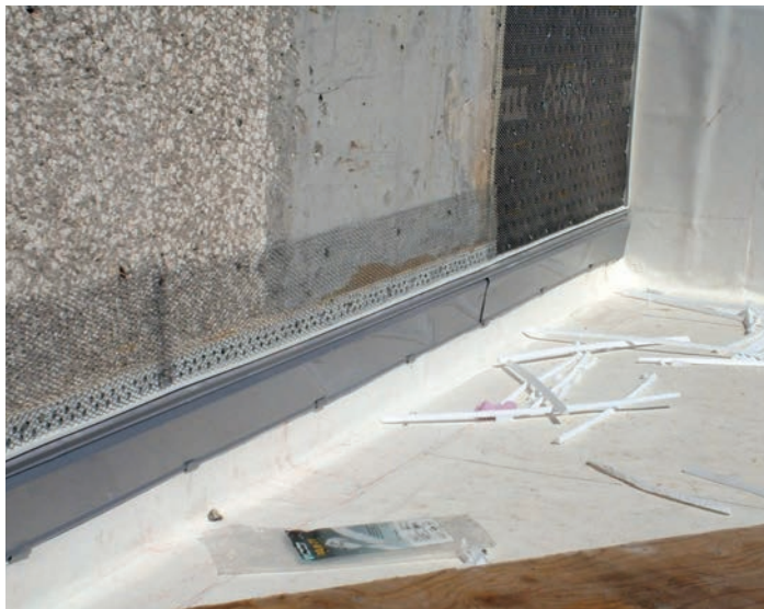
Wall flashing with metal counter-flashing
