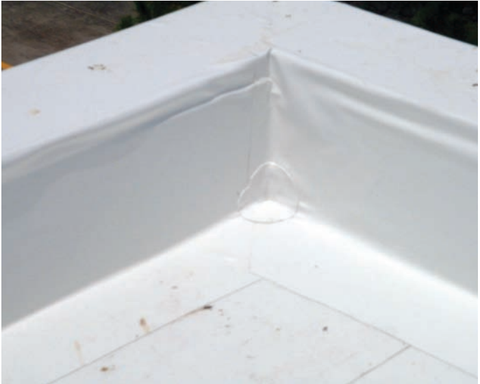
Pre-formed inside corner flashing
