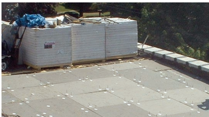
Mechanically fastened Flex insulation board
