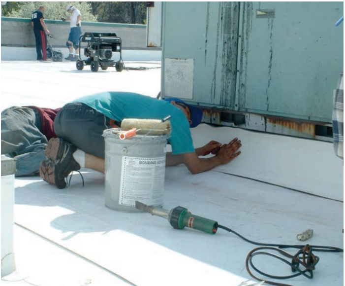
Flashing existing mechanical unit
