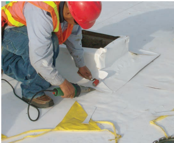
Hand welding a field-fabricated flashing
