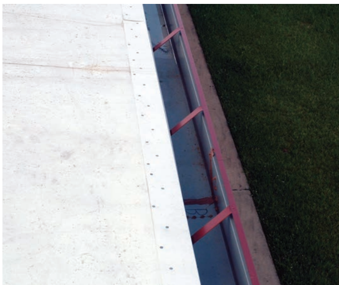
FlexClad™ metal drip edge, properly secured
