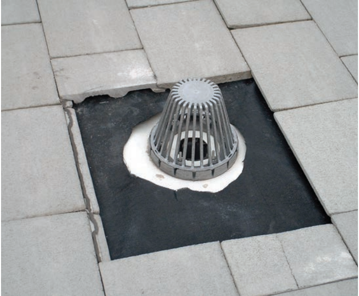
Pavers installed over properly flashed drain detail
