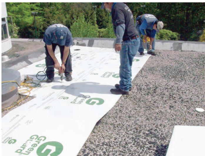
Placing Flex fan-fold GreenGuard re-cover board
