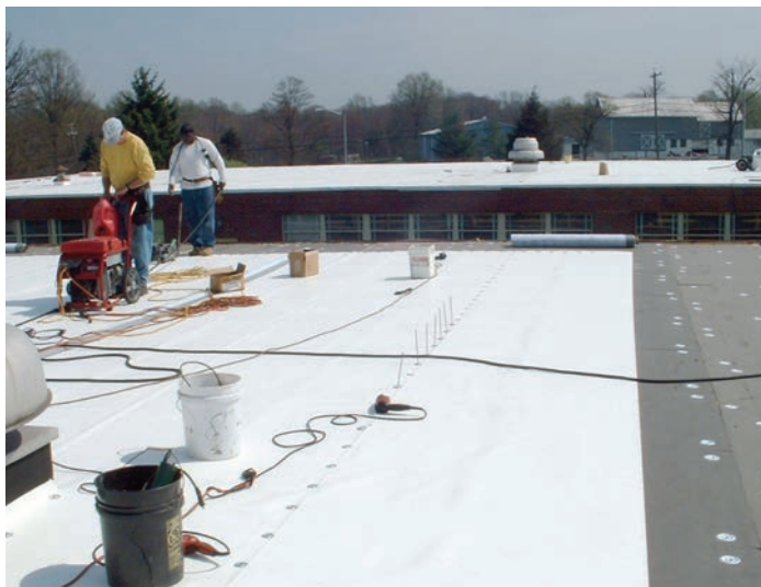
Mechanically fastened Flex TPO membrane
