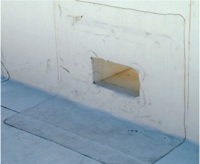
Through-wall scupper made of FlexClad™ Metal
