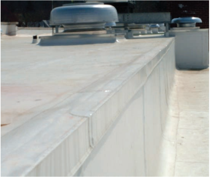
Flex Trim Strip welded to FlexClad™ metal and field membrane
