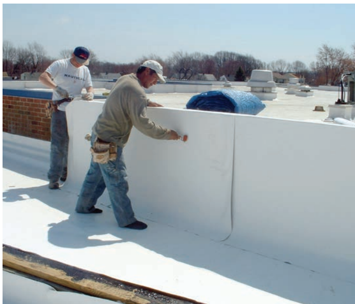
Rolling wall flashing into place
